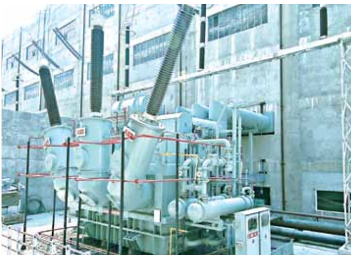
154 MVA, 11/420 kV Generator Transformer
