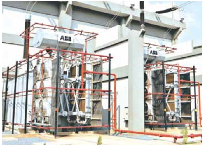
400/74.5/74.5kV HVDC back-to-back Converter Transformers
