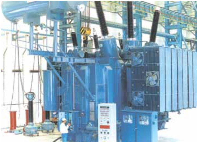
100 MVA 220/66 kV Power Transformer
