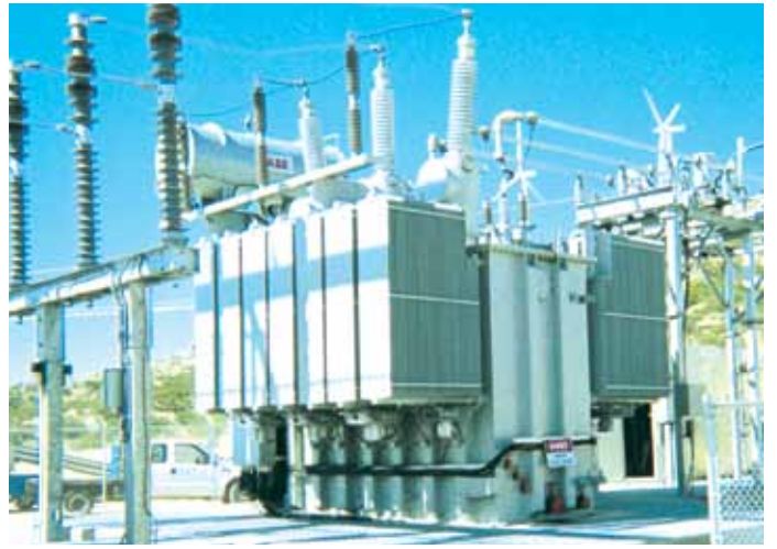
87.5 MVA, 138/34.5 kV Transformer
