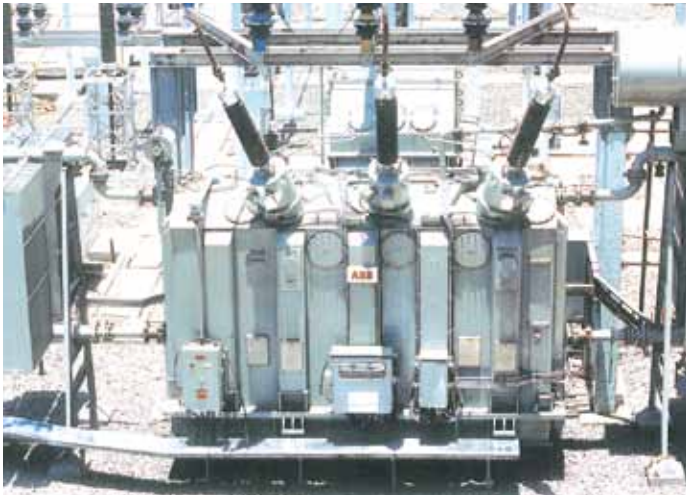
90 MVA, 110/34.5 kV Power Transformer
