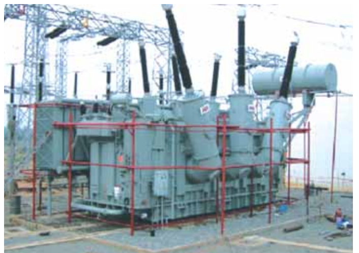
315 MVA, 400kV Auto Transformer
