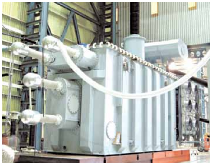
HVDC Converter Transformers
