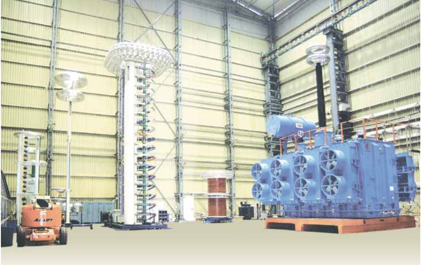
Testing facilities for transformer from 220kV to 765kV
