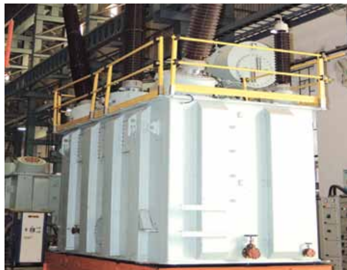
Shunt Reactors - 50-125 MVar 400kV class
